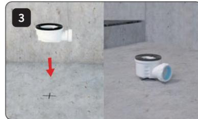
Check the product in the desired installation area. Sufficient space should be available.
