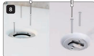
Tighten the 2 or 3 screws (depending on the version). Serrer les 2 ou 3 vis (selon la version).
