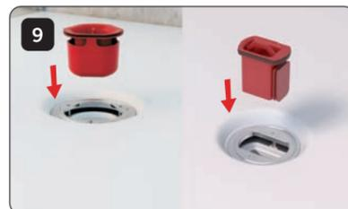
Insert the trap onto the shower waste outlet body. Check it correctly fits.
