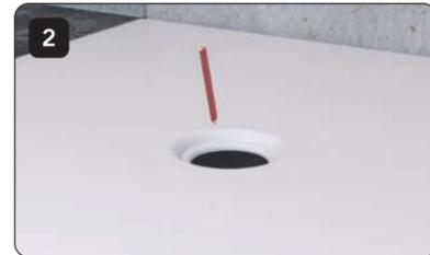
Choose the right model according to the shower tray hole (Ø52, 62 or 90 mm). Mark the position of the valve.
